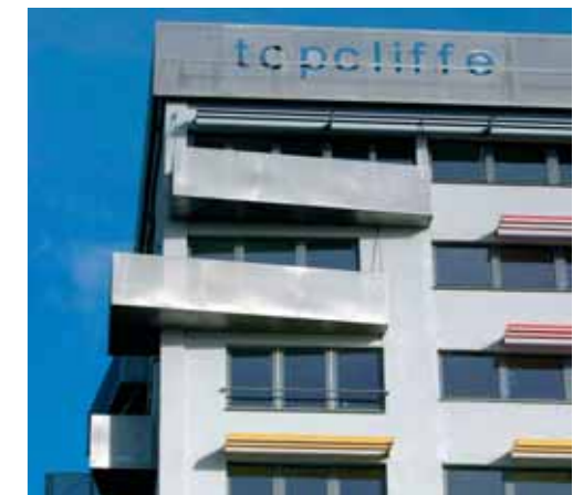
Topcliffe house has been transformed into a modern apartment block for the over 40s. It is one of only two of the original 34 tower blocks that now remain in Castle Vale.
