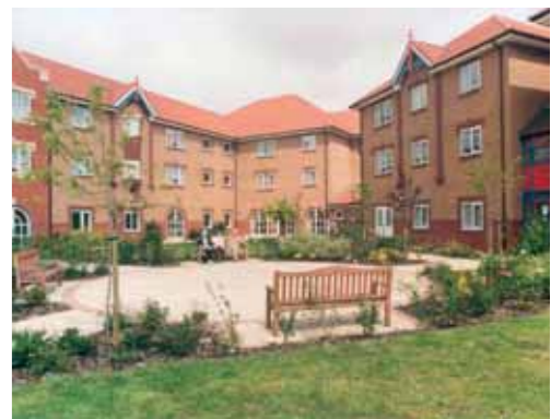
Phoenix Court extra care scheme replaced the warden scheme in Albert Shaw House, a 15 storey tower block demolished to make way for the redevelopment of the old Castle Vale shopping centre.
