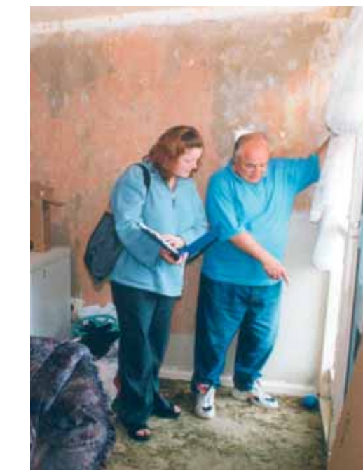
Resident liaison officers worked closely with tenants whose homes were being improved.
