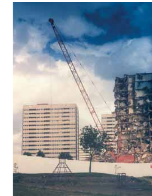
Demolition of the first four Centre 8 tower blocks.
