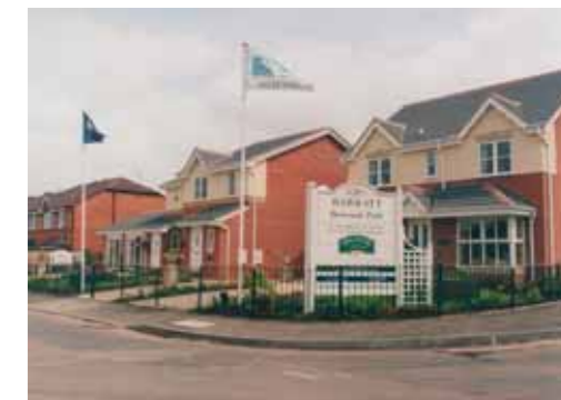
52 homes were built for sale by Barratt.
