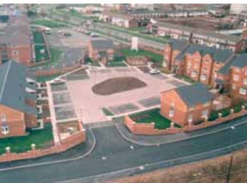
View of traditionally built homes on Farnborough Road, by Castle Vale swimming bath.
