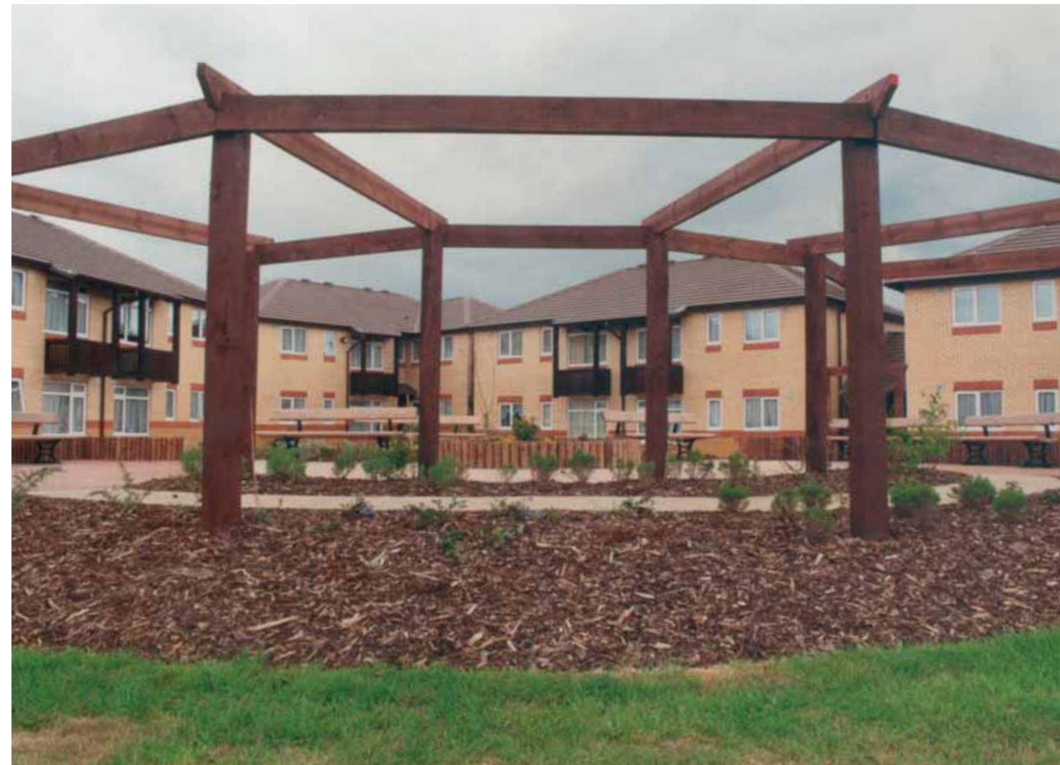
In 1995, 24 homes were built on the site of the former Albatross Pub.
