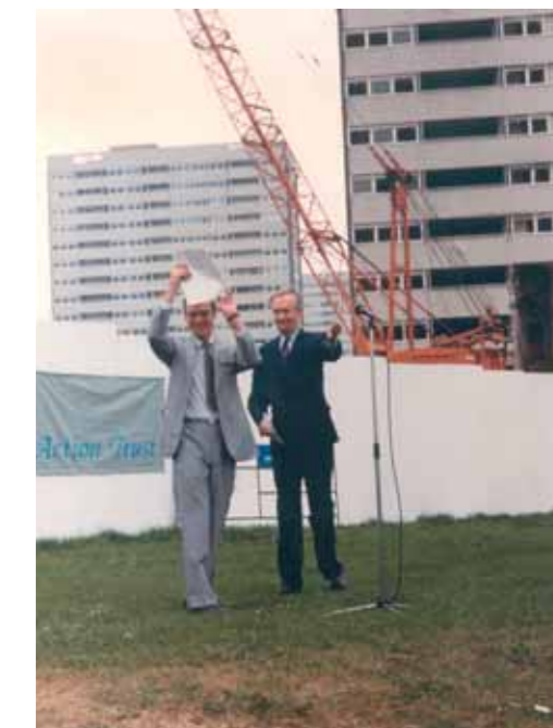
Chairperson of the Centre 8 Liaison Group Harry Poyner and HAT Chairman Richard Temple Cox, launch the start of demolition of the Centre 8 tower blocks in May 1995.
